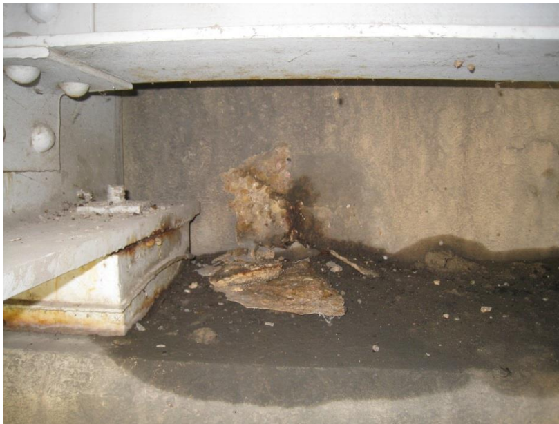
Figure 22. Typical isolated spall at abutment back wall, with exposed, corroded reinforcement (South Bridge Abutment 1 shown).
