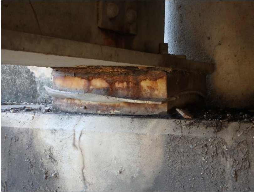
Figure 17. Corrosion of outermost bearing assembly, with deterioration/protrusion of lead sheet. Southeast corner of South Bridge shown.
