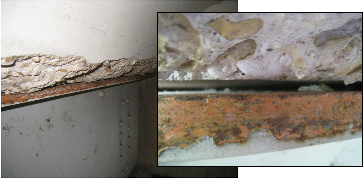
Figure 9. Typical gap at corner of North Bridge (southwest corner shown), with lack of apparent corrosion on girder top flange.
