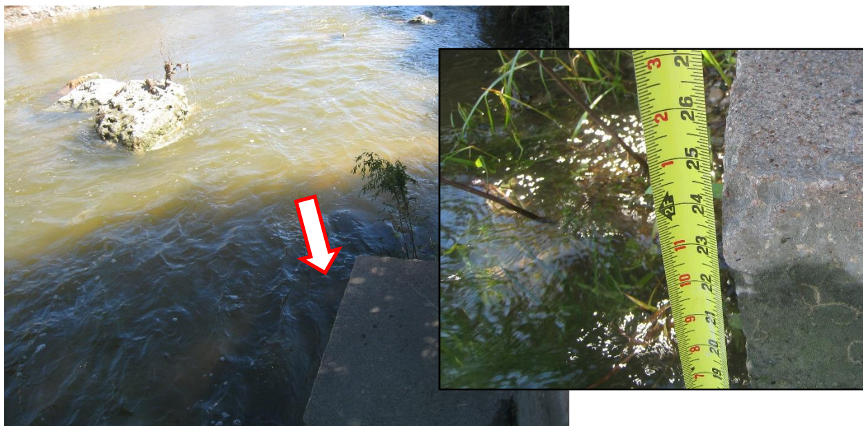
Figure 24. Scour at east end of South Bridge Pier 3, with concentrated water flow due to boulders in San Gabriel River.
