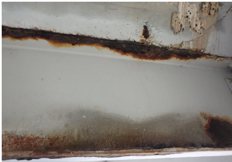
Figure 16. Typical pack rust formation at diaphragm top flange, with flange tip section loss.
