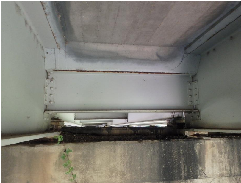
Figure 4. Typical diaphragm detailing (south end of North Bridge shown).
