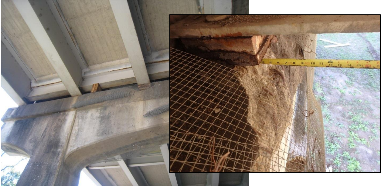
Figure 19. Large spall at South Bridge Bent 2.
