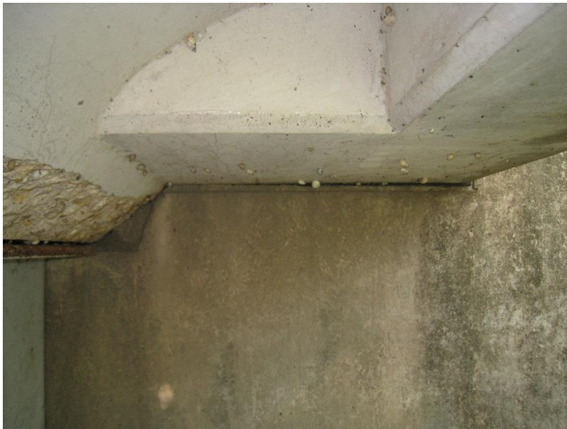
Figure 8. Typical movement at corner of North Bridge (southwest corner shown), with spalling along unreinforced haunch chamfer.
