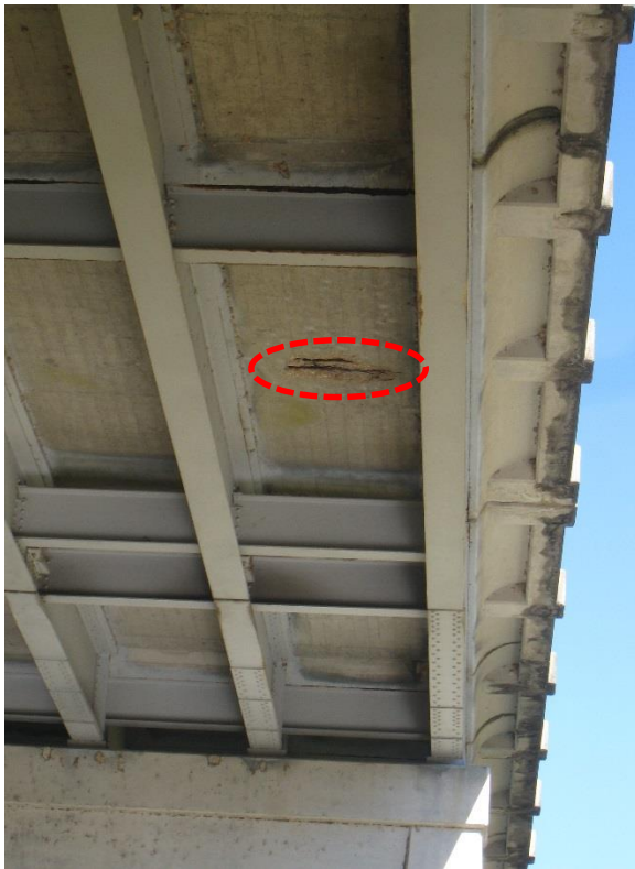
Figure 10. Typical, isolated deck soffit spall with two exposed, corroded bars (east side of South Bridge Span 3 shown).
