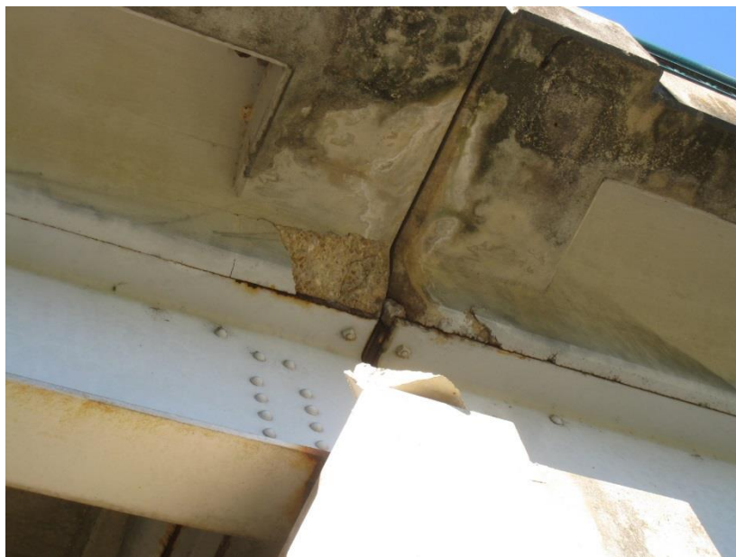
Figure 11. Typical chamfered haunch spall, with no visible reinforcement.
