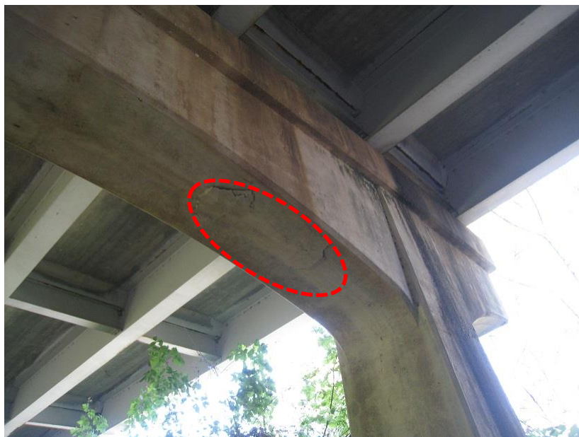
Figure 23. Isolated bent cap soffit spall (North Bridge Bent 2 shown).
