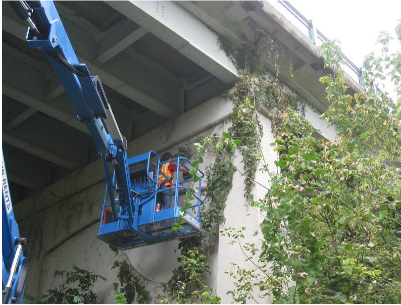
Figure 7. Use of 50-foot articulating boom lift to conduct non-destructive testing at North Bridge Pier 5.
