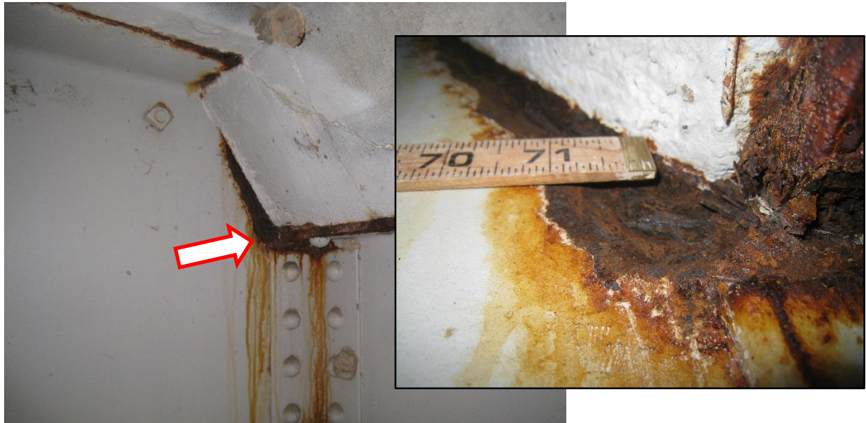
Figure 15. Moderate corrosion pitting of girder web at diaphragm connection, where diaphragm concrete is cast flush with steel (web section loss of approximately 1/8 inch). Interior face of outermost girder shown.
