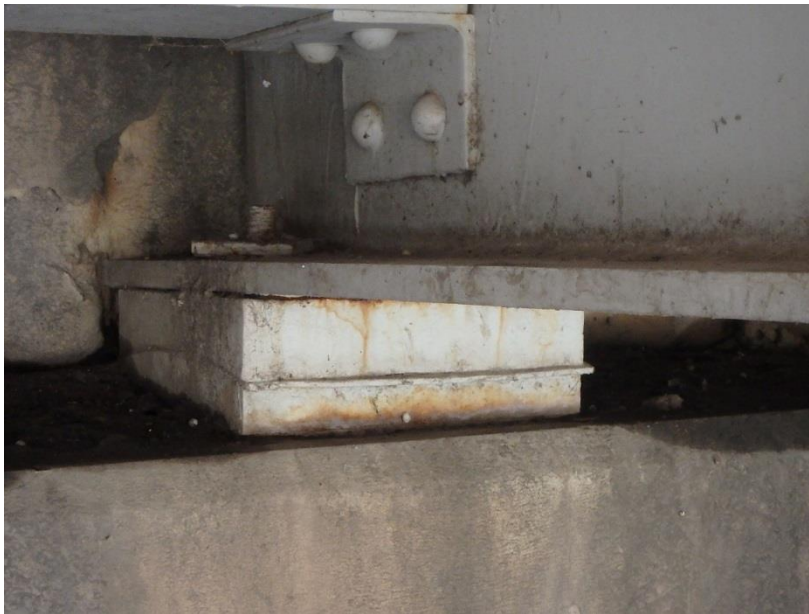
Figure 6. Typical bearing detail (south end of South Bridge shown).
