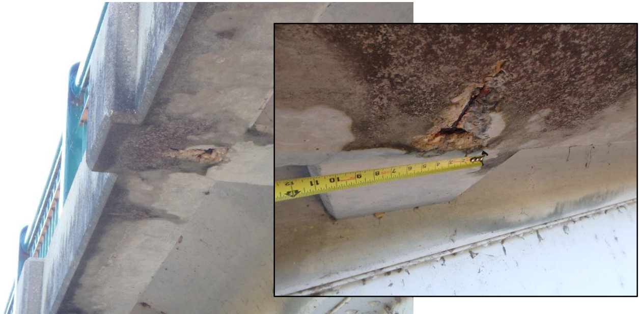
Figure 14. Typical isolated spall at base of pedestrian rail post, with exposed, corroded post base (northeast side of North Bridge shown).
