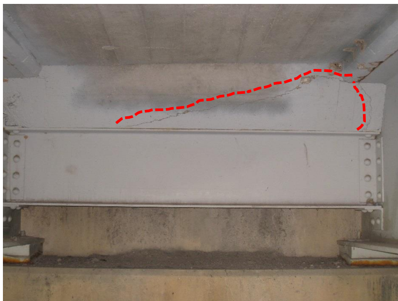
Figure 12. Typical cracking of diaphragm concrete, originating at reentrant corner created by girder top flange. Interior diaphragm with minimal corrosion shown.
