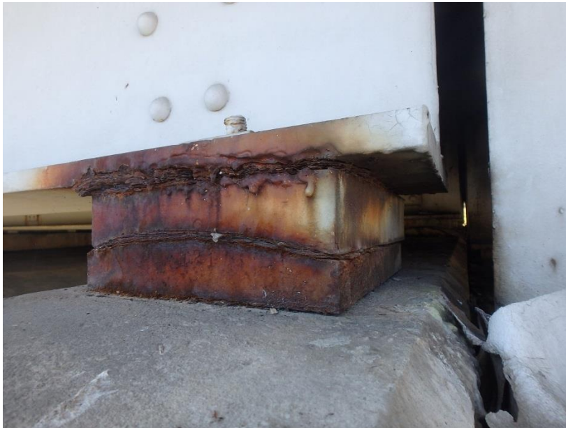
Figure 18. Pack rust formation at outermost bearing exposed to prolonged sidewalk drainage (east side of South Bridge Bent 2 shown).
