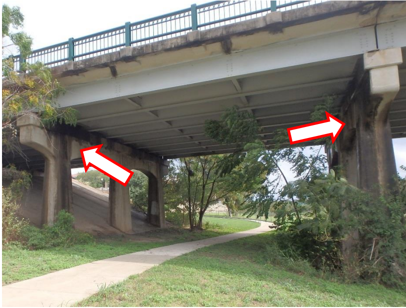
Figure 13. Typical leakage beneath expansion joints, with evidence of persistent moisture staining near exterior bent columns.
