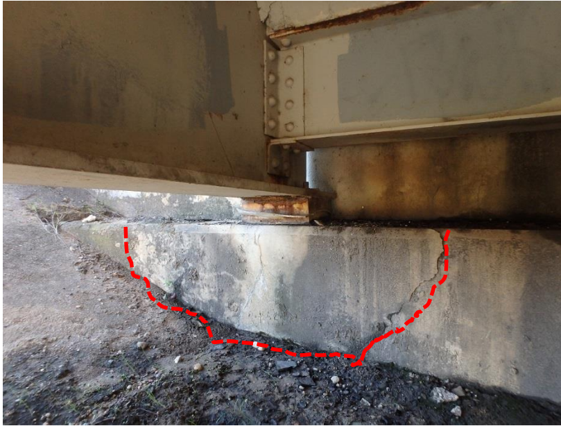
Figure 21. Delamination (insipient spall) at South Bridge Abutment 1, highlighted with red dashed line.
