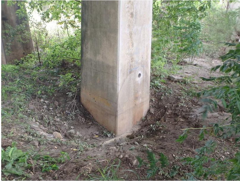
Figure 29. Core removed from South Bridge Bent 5 west face, from location exhibiting minimal surface staining (Core 11).
