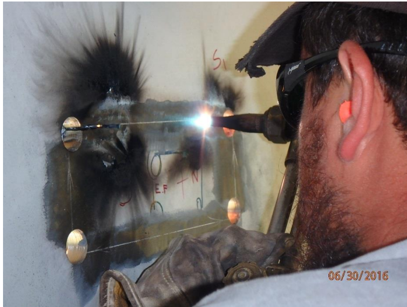
Figure 3. Ongoing torch-cut removal of steel web specimens.
