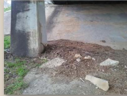
**Concrete** breaks off and drops from the bridge superstructure. Temporary netting or wire mesh has been installed in an area of concern for safety of trail users.
