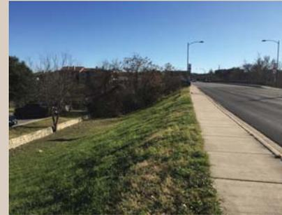
**Trail** is missing connections to Austin Avenue. **Sidewalk** on the bridge is four feet wide and does not meet standard accessibility and safety requirements.
