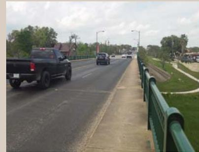
**Decorative Railing** on the bridge contained lead paint. The City performed lead abatement when the railings were repainted in 2009.
