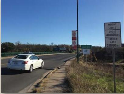
**Bridge Load Restriction** means loads that exceed the posting will accelerate deterioration but do not pose imminent danger. Examples of vehicles that exceed limits are loaded garbage trucks, and 18 – wheelers.
