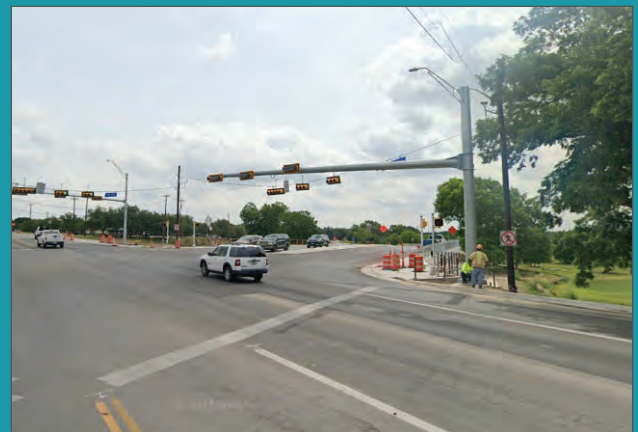
Weir Road/Northwest Boulevard
