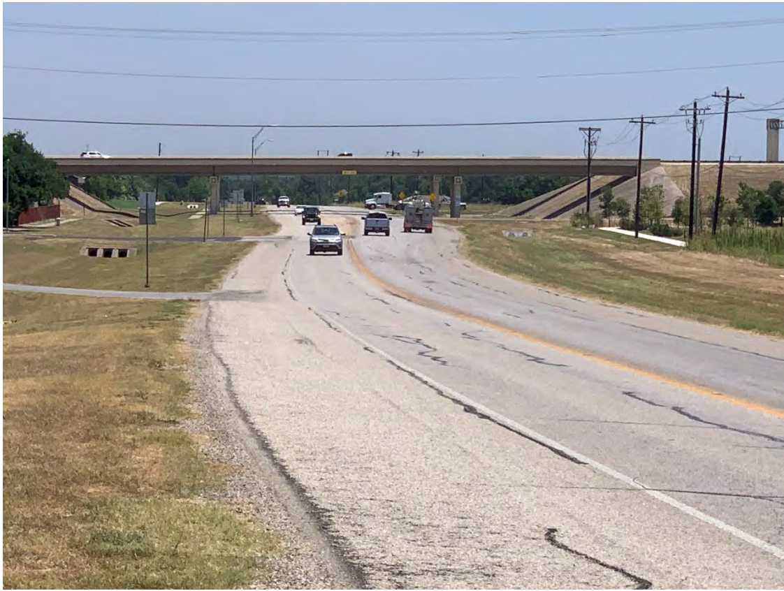
Overview of project area from 1,500 feet west of SH 130, facing northeast (Photo taken on 07/13/2023).
