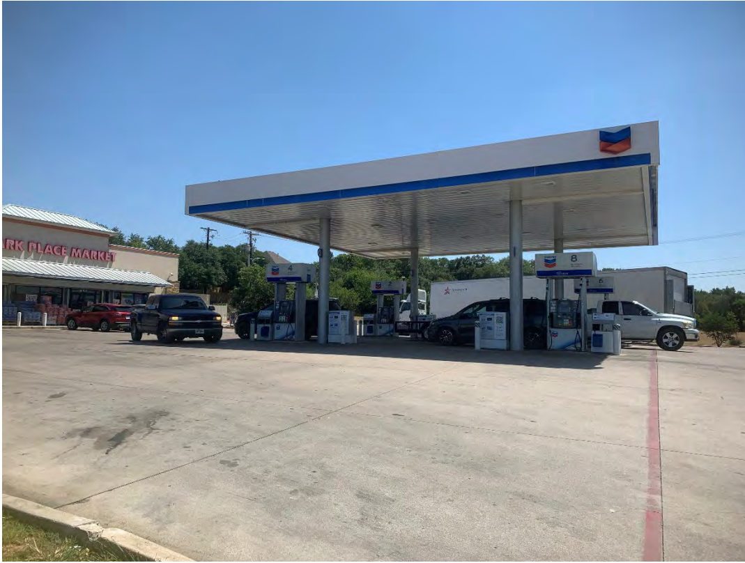
View UST site at Park Place Market/Chevron (Map Key 6), facing northeast (Photo taken on 07/12/2023).
