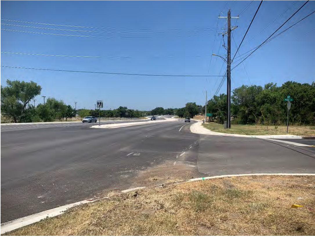
Overview of project area from Gann Street, facing northeast (Photo taken on 07/13/2023).
