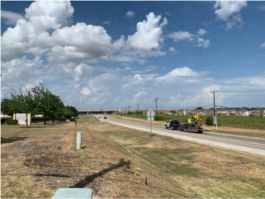
Photo 26: View of CR 152 and FM 971, facing east.
