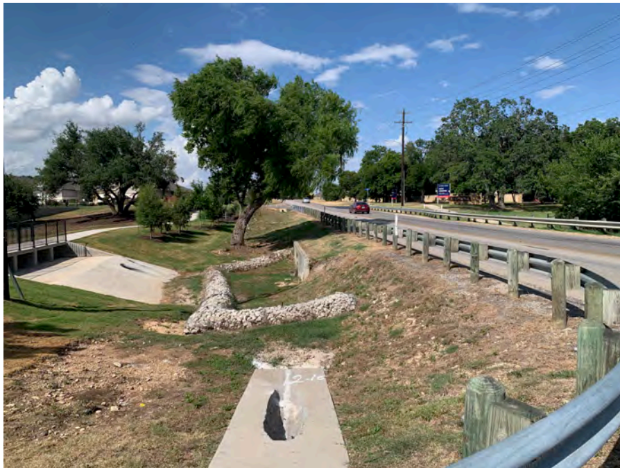
Photo 8: View of drainage structures adjacent to FM 971, facing northeast.
