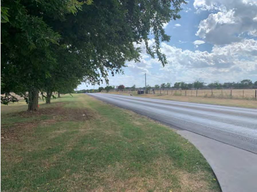
Photo 19: View of FM 971 from Deep Creek Road, facing southwest.
