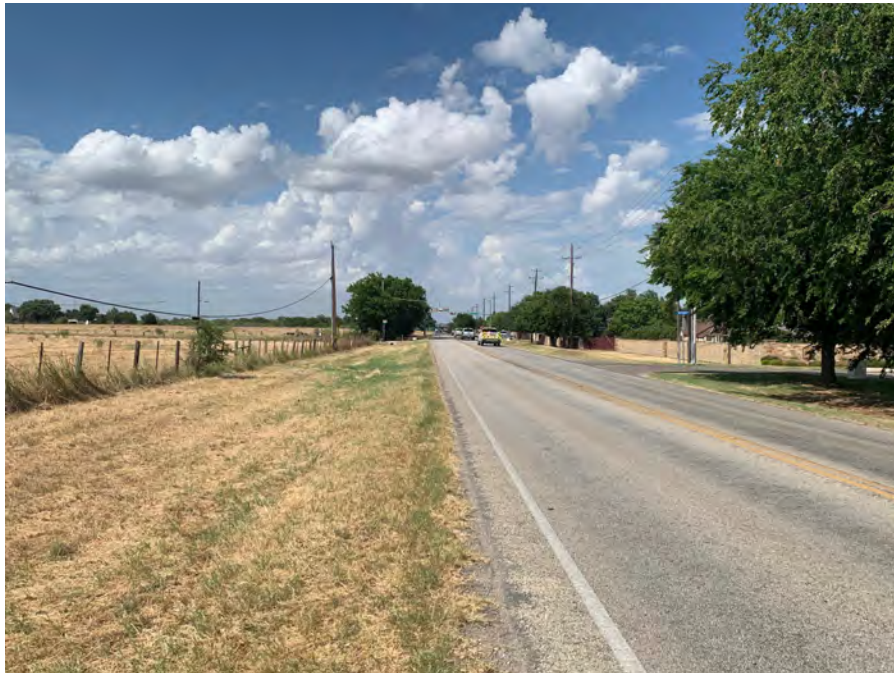
Photo 28: View of FM 971, facing northeast from south of Deep Creek Drive.
