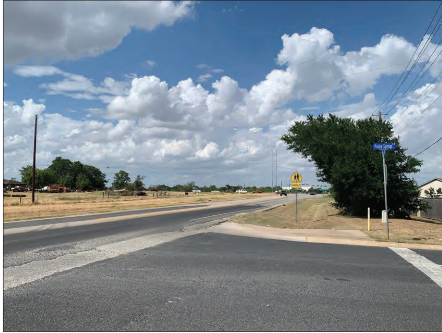
Figure 17. View of FM 971 from Prairie Springs Lane (Facing Northeast)
