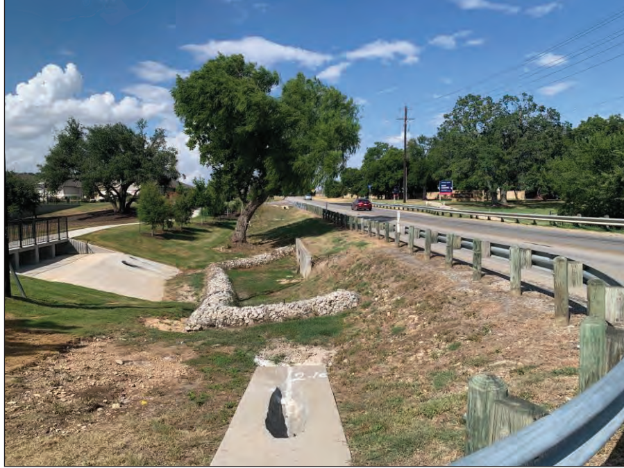
Figure 25. View of Drainage Structures Adjacent to FM 971 (Facing Northeast)
