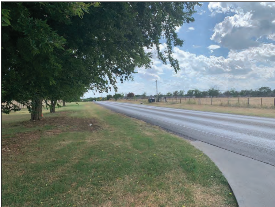
Figure 14. View of FM 971 from Deep Creek Road (Facing Southwest)
