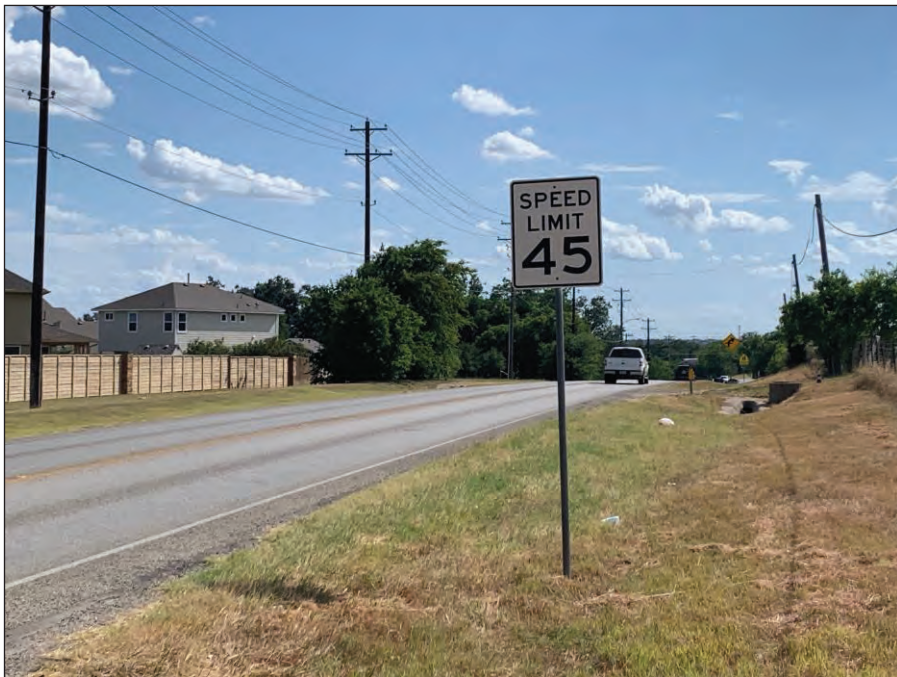
Figure 24. View of FM 971 near Parkside Crossing Residential Subdivision (Facing Southwest)
