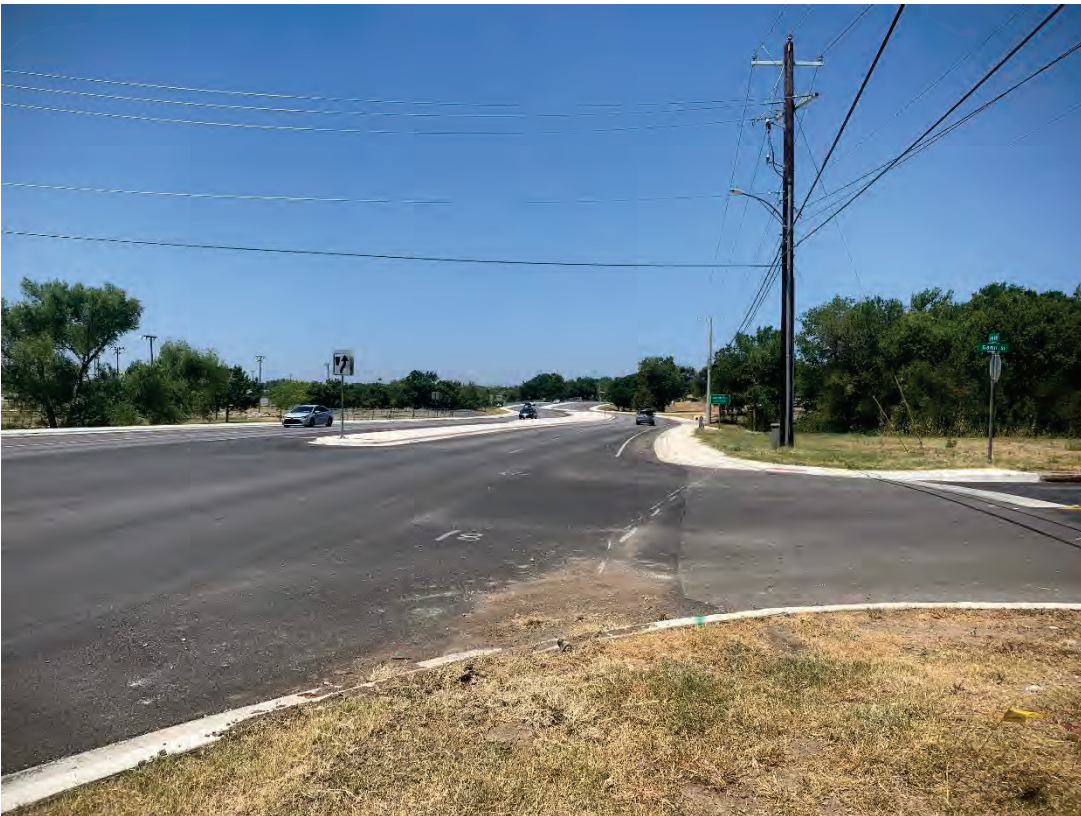
Overview of project area from Gann Street, facing southwest (Photo taken on 07/13/2023).
