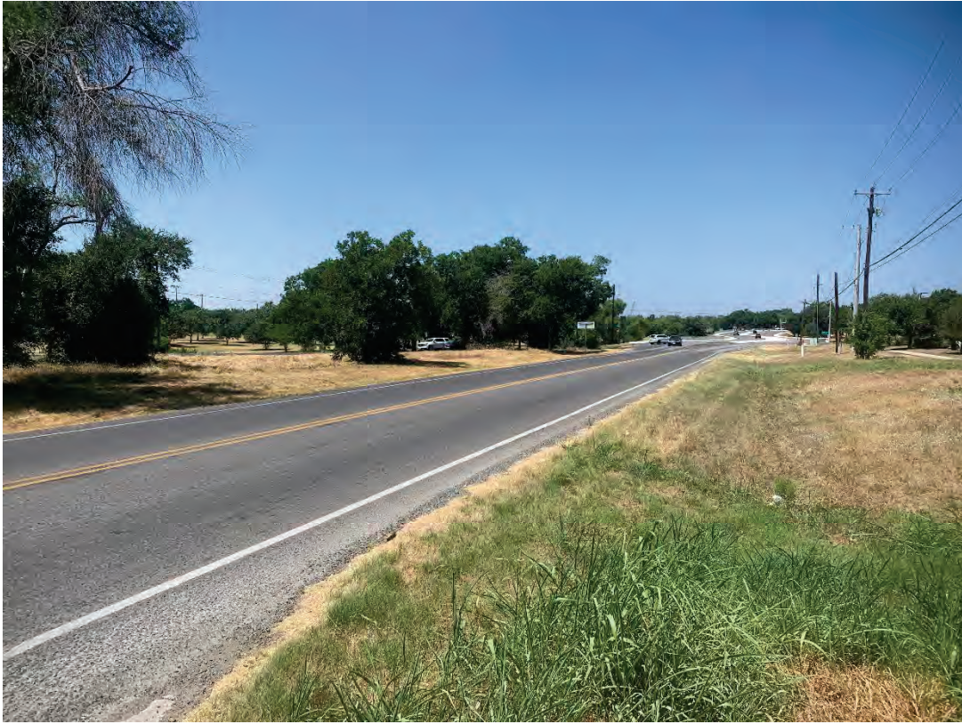
Overview of project area from 1,000 feet east of Gann Street, facing southwest (Photo taken on 07/13/2023).
