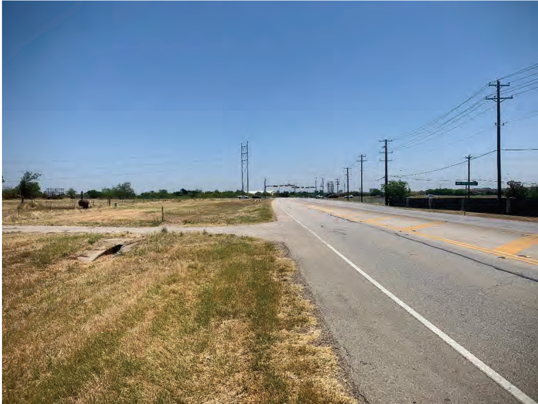
Overview of project area from 2,000 feet west of Inner Loop, facing northeast (Photo taken on 07/13/2023).
