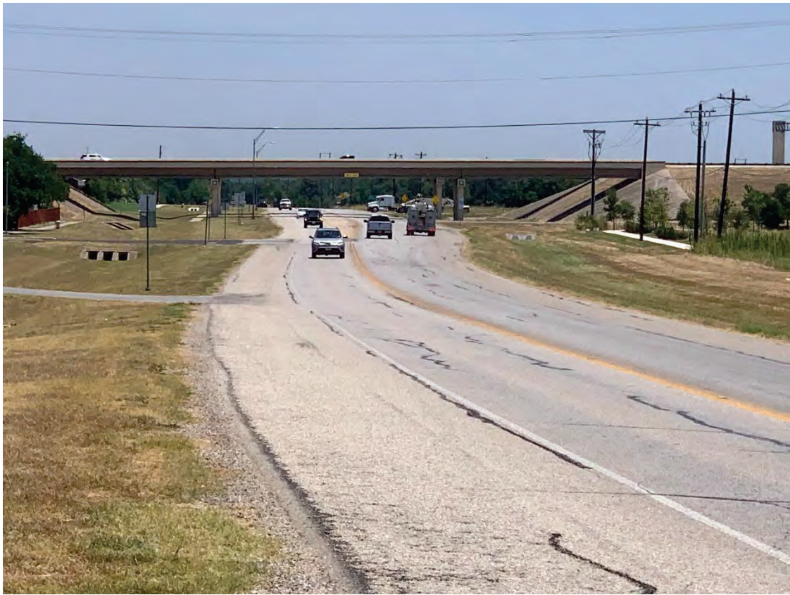
Overview of project area from 1,500 feet west of SH 130, facing northeast (Photo taken on 07/13/2023).
